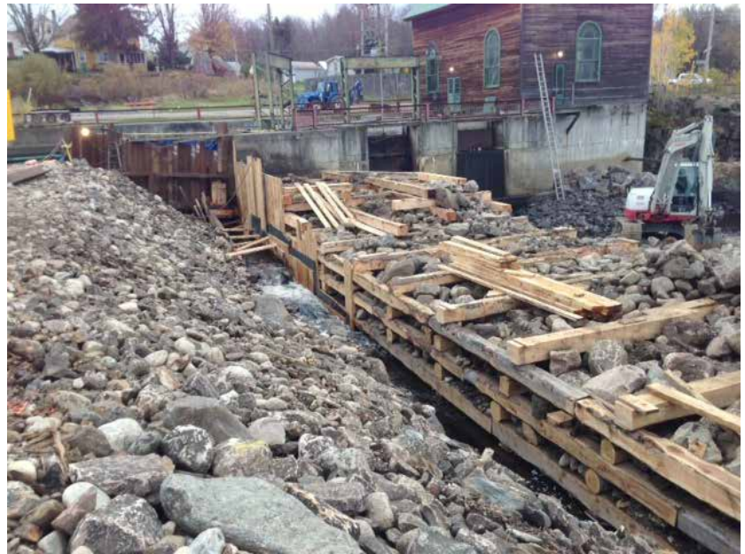
Figure 44: Lumber Crib dam under construction
