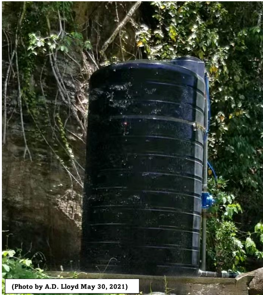
Figure 18 Temporary water storage at Coulibistrie. Water is abstracted from the lower section of the Watershed
